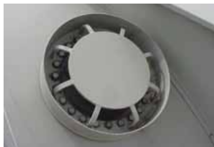
Figure 1- Typical Turbine Rupture Disc Housing
