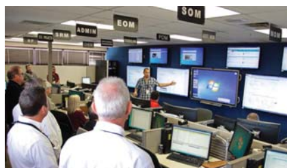
Updated Unit 2 Outage Control Center Video Wall.
