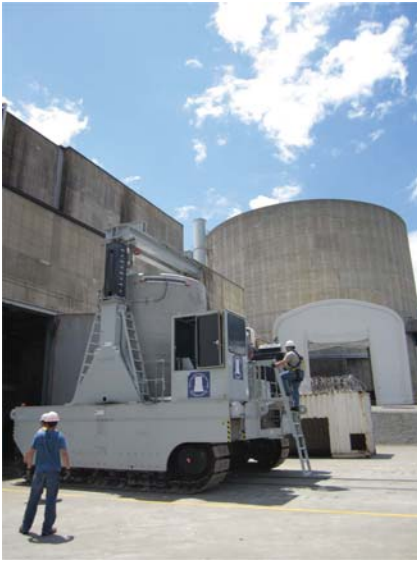
MAGNASTOR® VCC Docked with Vertical Cask Transporter.
